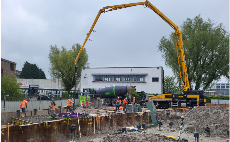
Urban Mine concrete with 100% FreeGravel 60% FreeSand and Freement being casted for the Mama Shelter Hotel in Amsterdam (Photo: TBI and Urban Mine)
