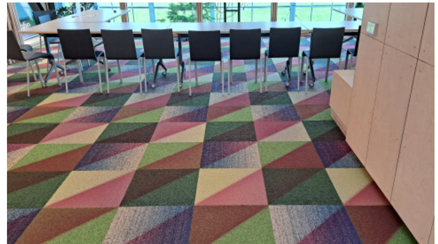
Interior finishes like these carpet tiles were sourced from other buildings and reused/repurposed for the Biopartner 5 building (Photo: Bas Horsting)
