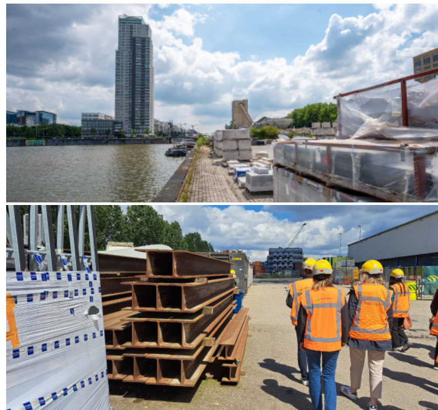
View of Ship it facility in Brussels (Photos: Fabio Bayro Kaiser)
