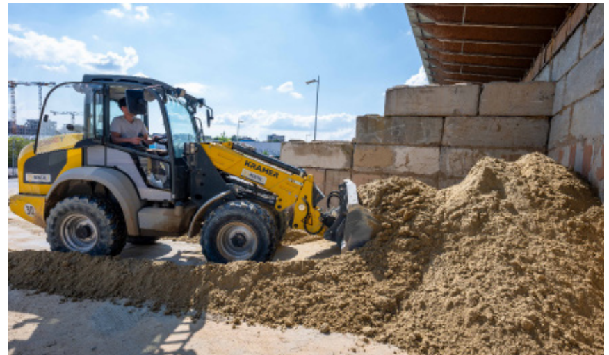
On-site tour of BC Materials facility in Brussels (Photo: Fabio Bayro Kaiser)
