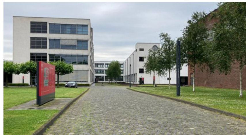
View of the modernist (Bauhaus) style industrial estate Mies van der Rohe Campus (Photo: KREFELD BUSINESS)
