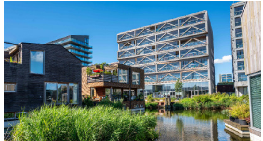
PATCH22 Building in Buiksloterham, Amsterdam (Photo: Fabio Bayro Kaiser)
